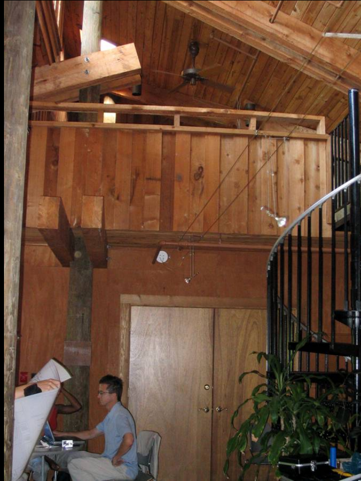
Loft space in the dining hall: view looking west.
